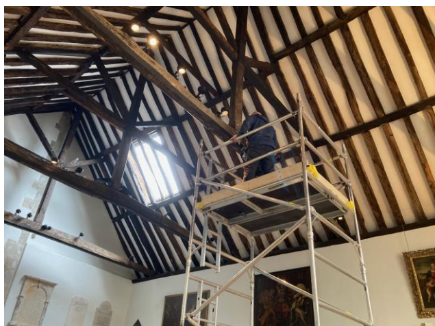
Electricians at work
